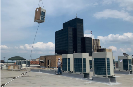
Rooftop HVAC Condensers
